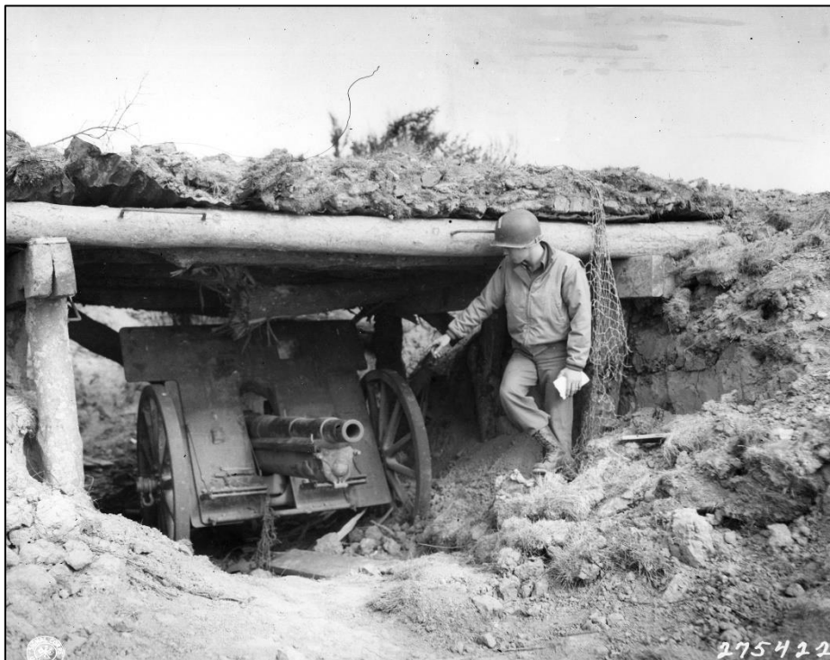
The Skoda 7.65cm FK17(t) Feldkanones at WN-74 sited to fire along OMAHA Beach [SC-275422]
