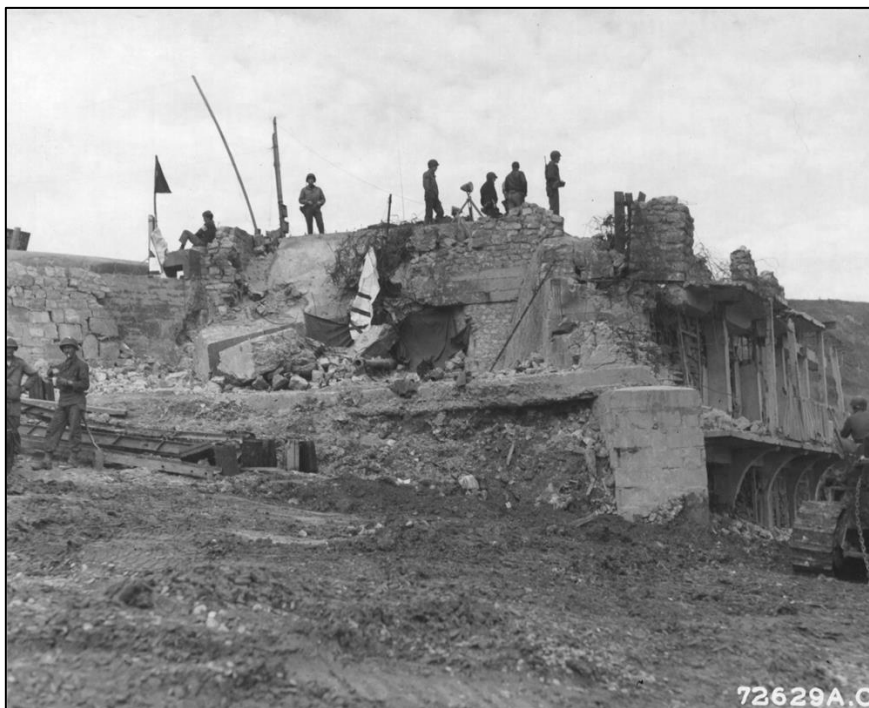
The remnants of the hotel can be seen in front of the Regelbau H667 casemate housing the 8.8cm Pak 43/41 at the seaward end of the D-1 Vierville draw. [72629-AC]
